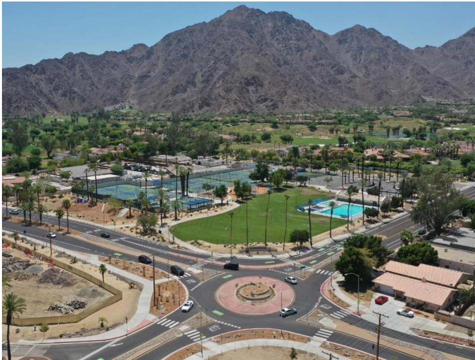
Figure 3-22. La Quinta Village Complete Streets Project
