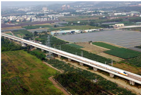
Taiwan’s high-speed rail system operates on elevated structure to accommodate land use.
