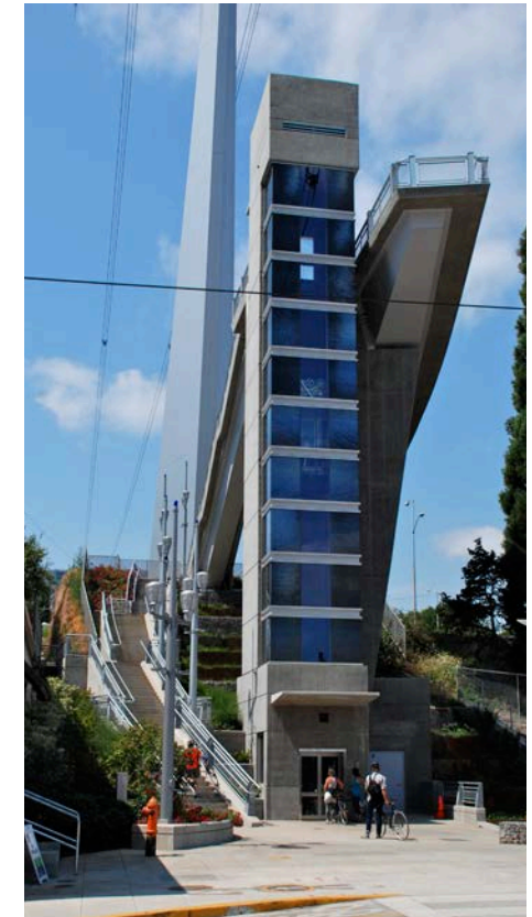
Elevator at Gibbs St Pedestrian Bridge; Portland, OR
