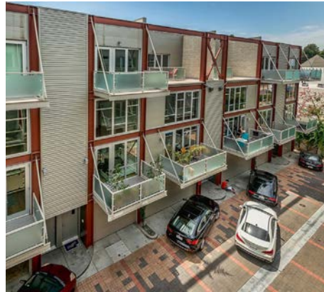
Tuck-Under Parking Court as a shared amenity
