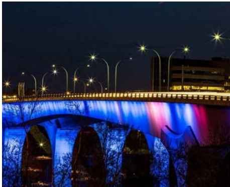
35-W Bridge; Minneapolis, MN
