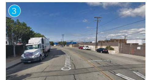
Auto-oriented road along Commercial Avenue
