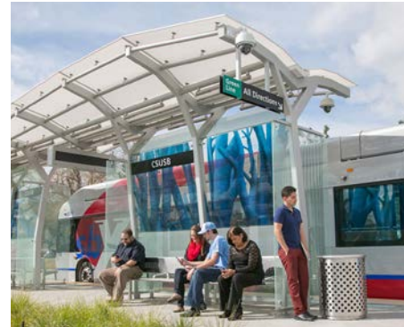
sbX Transit Shelter, San Bernardino, CA
