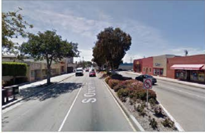
Existing Condition: Two very wide, fast vehicular lanes northbound and southbound, armored raised medians with Australian Paperbark trees, no on-street parking, and sidewalks in most cases either obstructed and lifted by very large Ficus trees or lacking street trees entirely.
