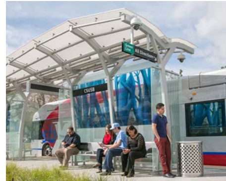
sbX Transit Shelter, San Bernardino, CA
