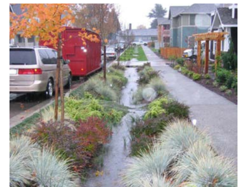
Bioswale, Seattle, WA
