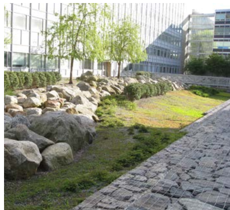
Bioswale, Boston, MA
