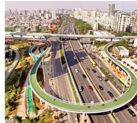
Bicycle Bridge; Xiamen, China
