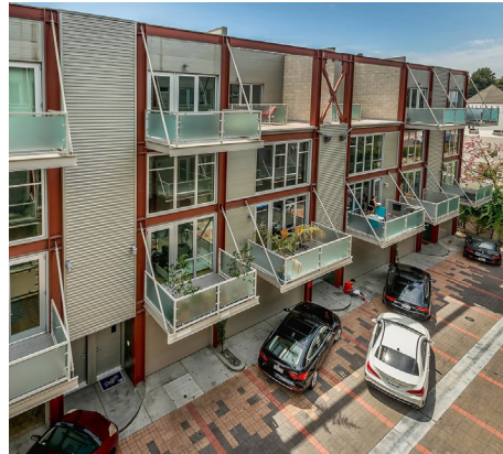
Tuck-Under Parking Court as a shared amenity
