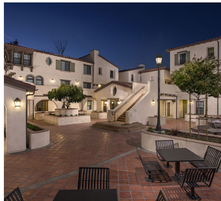
Terraces at Santiago, Santa Ana, CA
