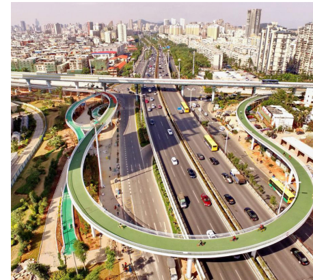
Bicycle Bridge; Xiamen, China
