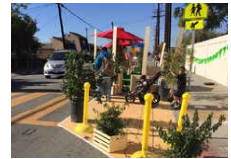
A bulbout was added to an existing mid-block crosswalk on Elizabeth Street to enhance pedestrian safety.
