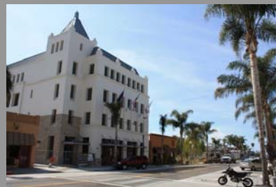
Infill Development on California St. Source: Ventura County Start
