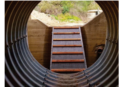
Retrofitted culvert under Route 118 in Ventura Country
