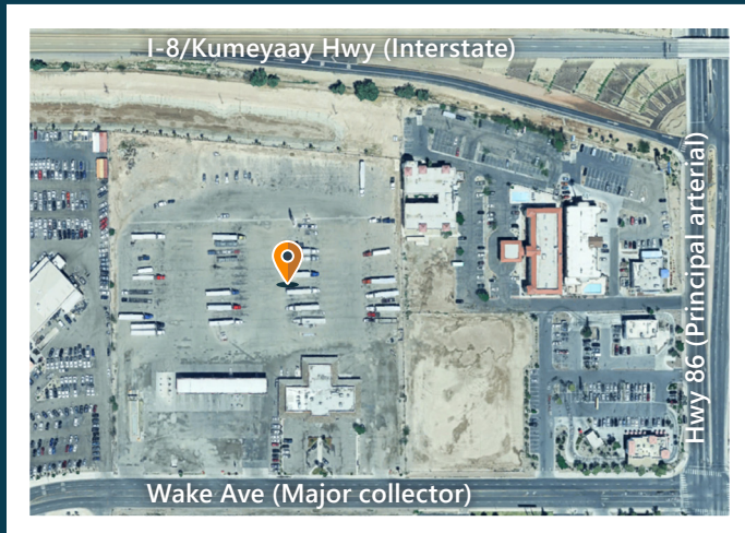
SITE AERIAL VIEW
