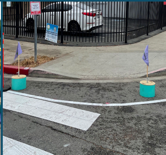
By tightening intersection curb radii, curb extensions enhance safety by encouraging slower vehicle turning speeds and creating shorter crossings for people walking.
