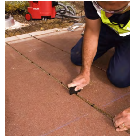
Installation of embedded piezoelectric strips
