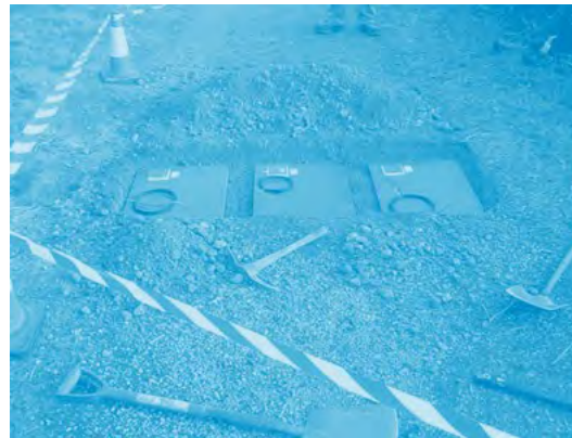
Pressure pads on unpaved path before being covered
