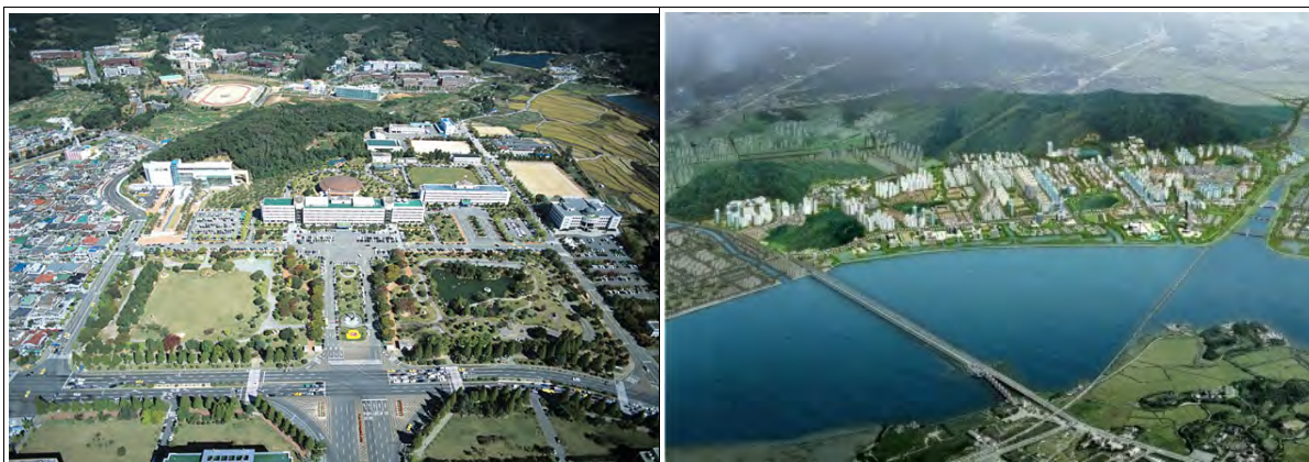
Figure 1. Domestic practices on the New Provincial Capital (Gyeongsangnam-do provincial office, Jeollanam-do provincial office) plans
