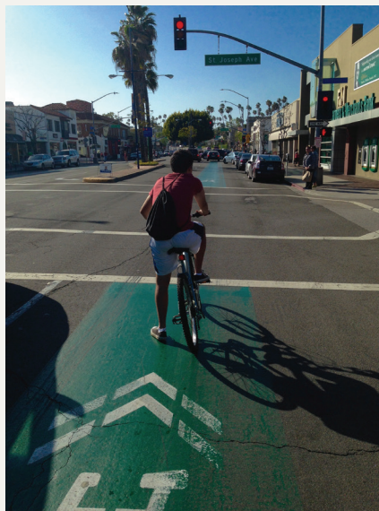
2nd Street Sharrows help keep bicyclists out of the door-zone and encourages bikes and cars to safely share the street (Source: Steer Davies Gleave)
