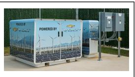
Stationary battery energy storage systems like this power bank are able to store energy generated from renewable sources and release it when needed.
