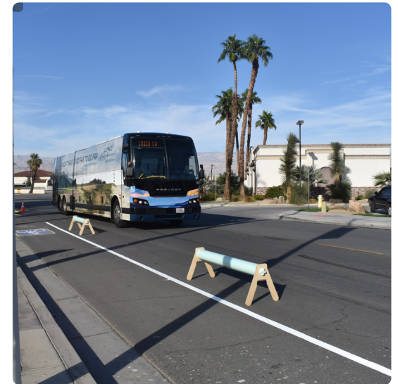
Lane partially closed for bike lane element
