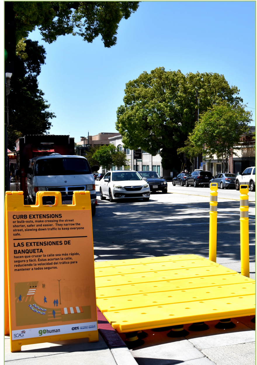
Kit of Parts Activation: Activate Fair Oaks curb extension
