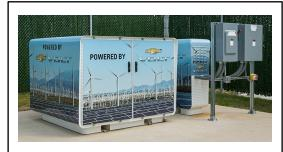
Stationary battery energy storage systems like this power bank are able to store energy generated from renewable sources and release it when needed.
