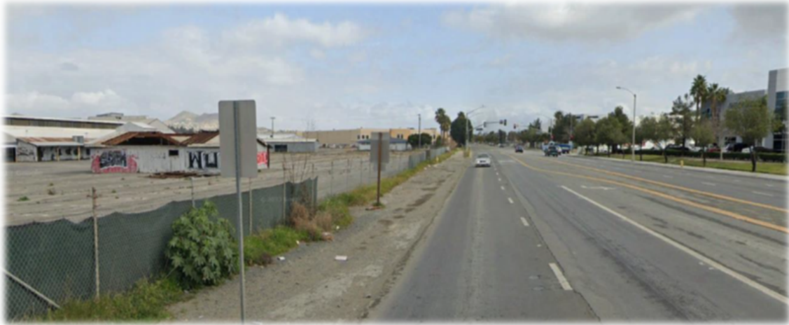
Figure 4: Missing Sidewalk & Bicycle Lane Northside of Magnolia Avenue
